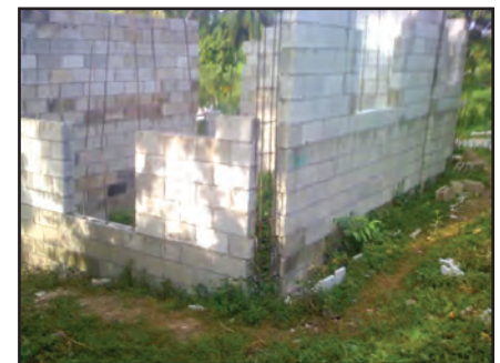
Ancient Bongo Issacs gates in progress
